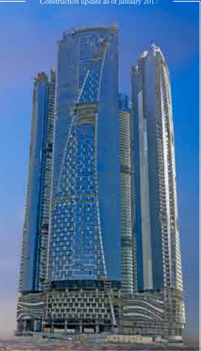
Construction update as of January 2017
